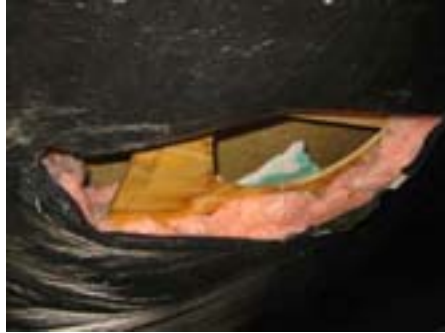
Figure 2-12 Bottom board hole in single section home
