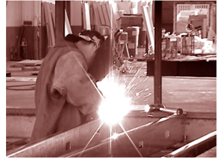
Rubber mallets and welding torches are standard equipment at QHP.
