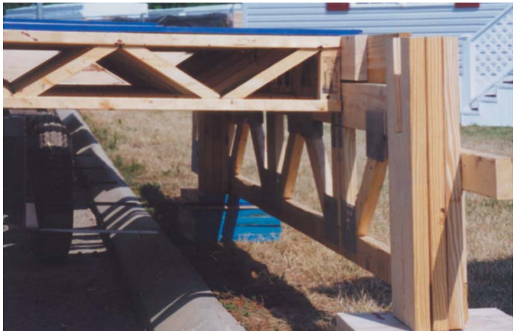
Treated stem wall of a Lindsay Unified Floor design.
