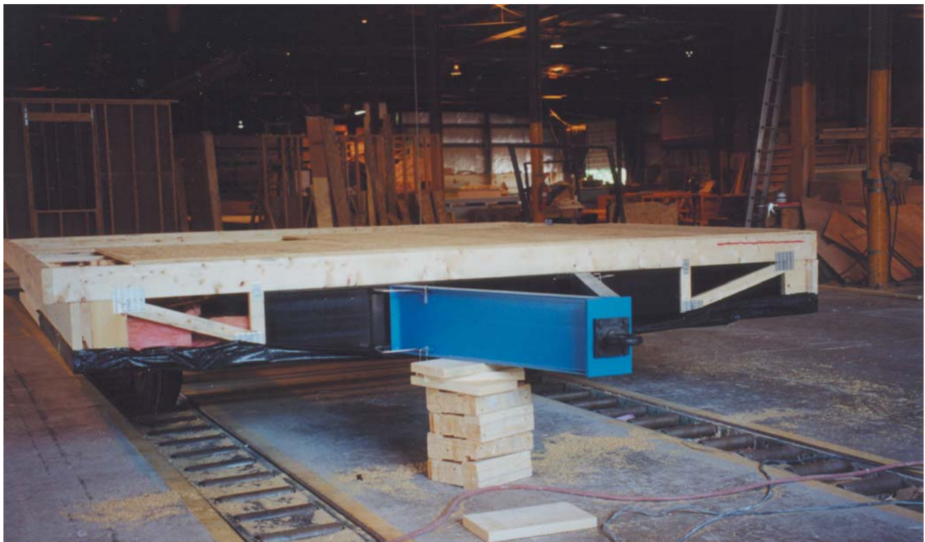
This Lindsay Unified Floor System uses a new "three-minute hitch" that saves on crane time.
