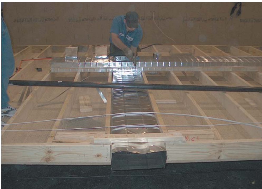
Manufacturers using the joist duct systems and mastic for duct sealing had a head start toward achieving ENERGY STAR efficiency targets.
