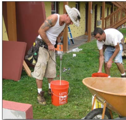
The adhesive is mixed on-site.
