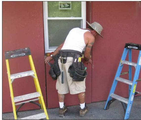
The panel below the window is installed.
