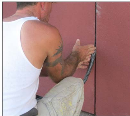
Backer rod is installed in the joints between panels.
