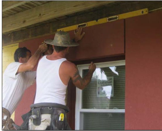
A panel over a window is placed and leveled.
